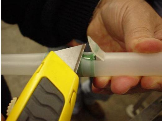
Make sure that the Perforator drilling of the pipe is not scratching the dripper pool.
